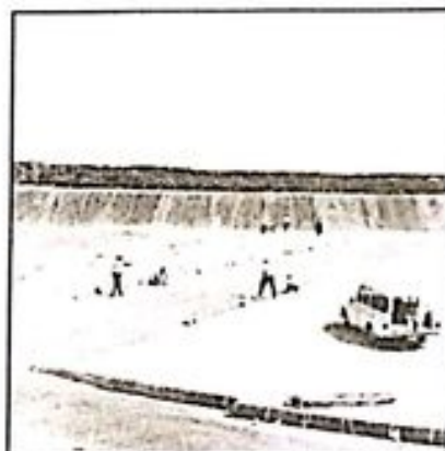
LINING ONE RESERVOIR WITH SYNTHETIC RUBBER
